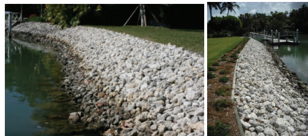
Figure 2-2. Rip Rap is rock used to armor [10]
